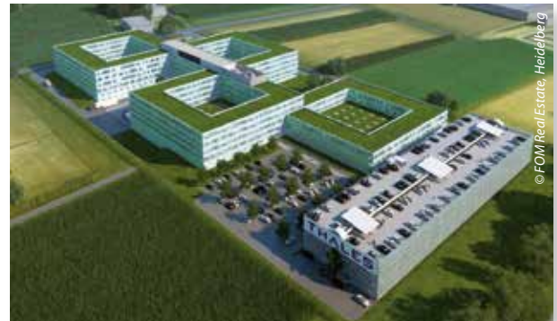
The corporate headquarters of Thales Deutschland GmbH in Ditzingen was completed in 2014. The Modbus-interface allowed the OPP-SENS ® sensors from Oppermann to be seamlessly integrated into the DDC automation systems from Schneider and Wago.
